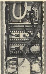
Elimination of fixed rack harnesse means components are completely in dependent for optimum flexibility.
